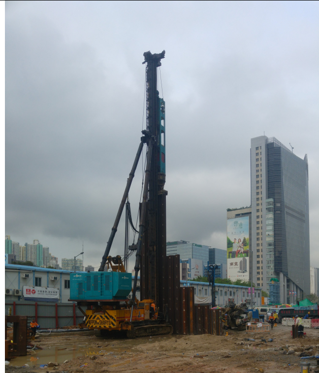
Site inspection photo of 4 th May 2017
