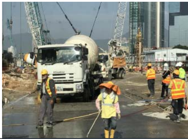
Wheel washing at the site entrance was provided on 7 December 2016.
