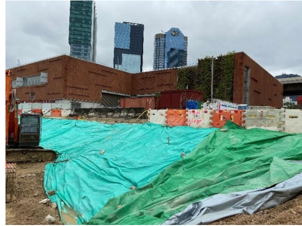
Photo 7 – Covering excavated area with tarpaulin sheet
