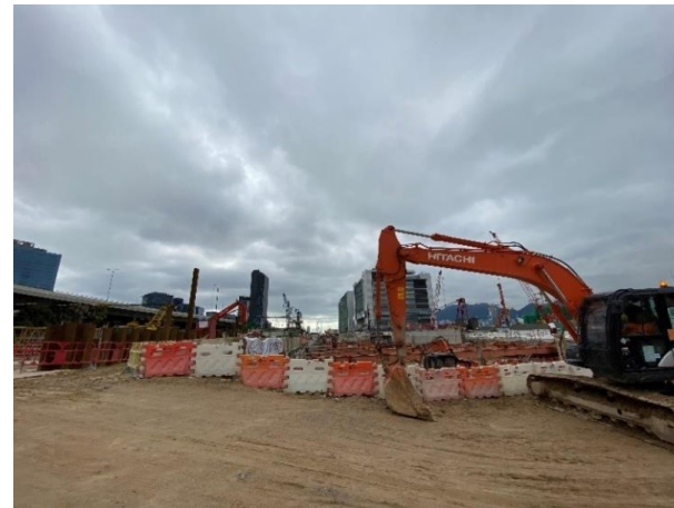
Photo 9 – Watering of unpaved road
